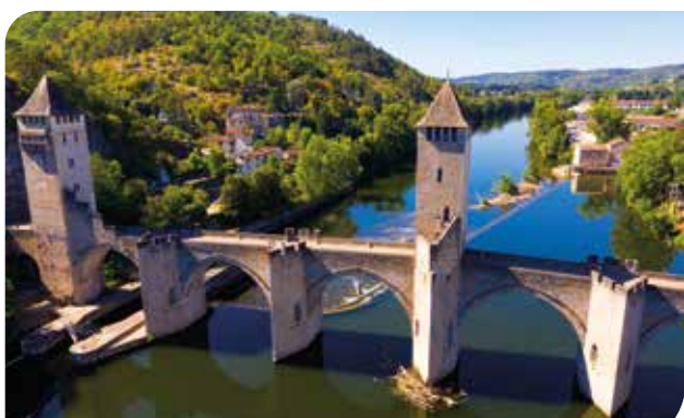
Valentré bridge, Cahors ©Getty Images/Jack F
